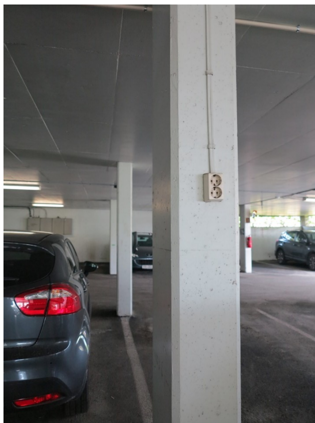
Figure 3-4 Prior to the installation of charging units, power sockets intended for engine heaters were used to charge electric cars. Following the installation of the charging system, a ban has been placed on the charging of cars via power sockets.
