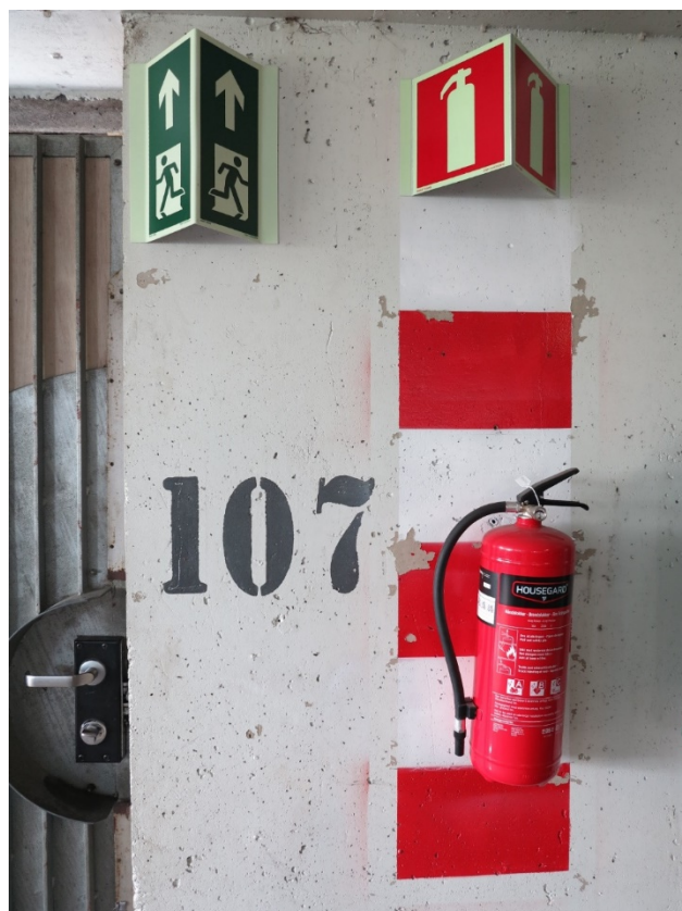
Figure 3-9 The labelling of escape routes and fire extinguishers was improved following a previous fire safety inspection. There are four portable fire extinguishers available on each level.
