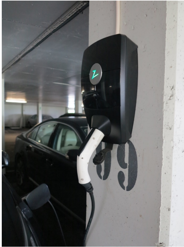
Figure 3-7 All of the charging units in the garage are from the same supplier and form part of the dynamic charging system.
