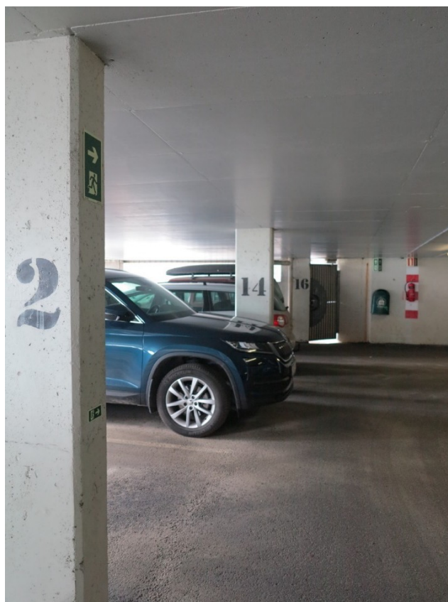
Figure 3-10 Escape routes are marked in several places in the garage.
