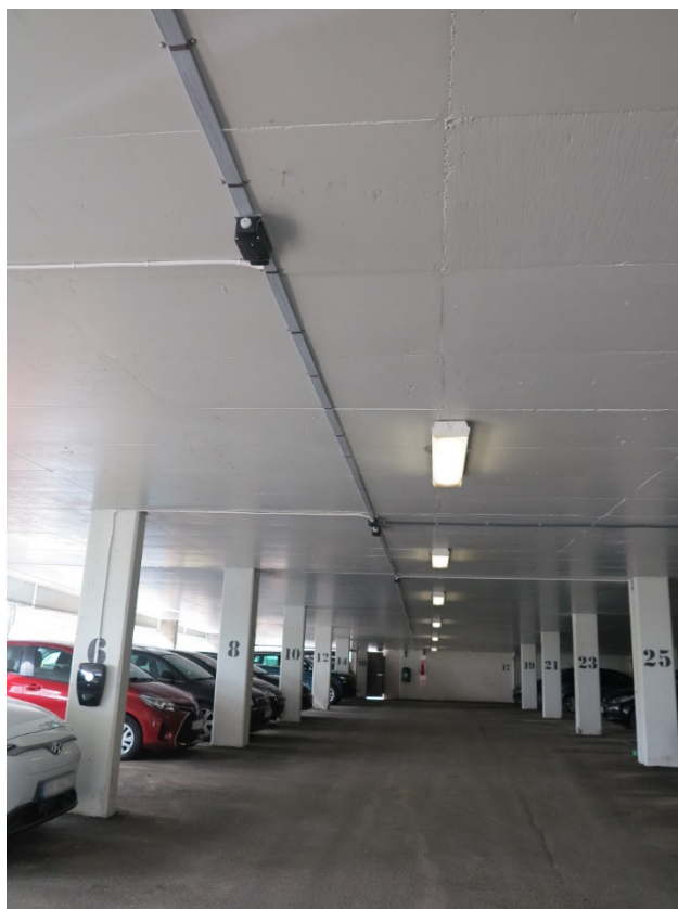
Figure 3-5 Two main cables on each floor supply power to the charging units (flat cable in the ceiling, middle of picture). Cables are laid from the main cable to the charging units. The electrical system has capacity for all of the parking spaces to be connected to the charging system. Car owners are free to choose whether they want to connect to the system, but need to connect to the system if they wish to charge a vehicle in the garage.
